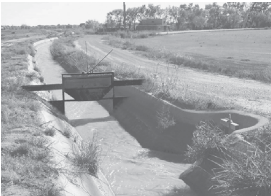
The metal structure on the left is a check. When it is closed the water in the high-line canal or lateral builds up to a level that will flow through the turnout, shown at lower right, into a farm field or smaller ditch.
